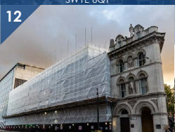
Holborn Viaduct EC1A 2AT
